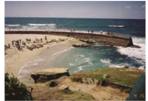
La Jolla Children's Pool Beach Management and Water Quality improvement- La-Jolla, California
